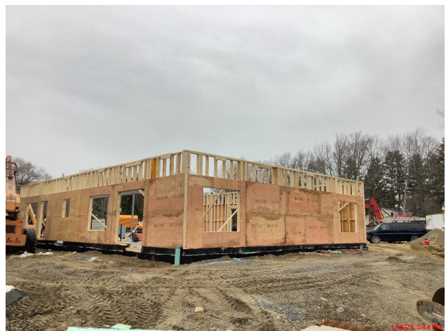
Some of the completed exterior framing on the Barn.
