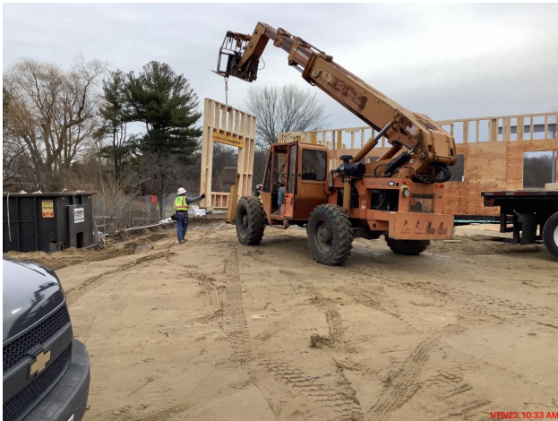
Putting the panels that will hold the walls in place.
